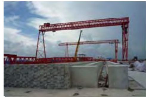
Construction sites of Coastal Expressway (Shenzhen Section)
